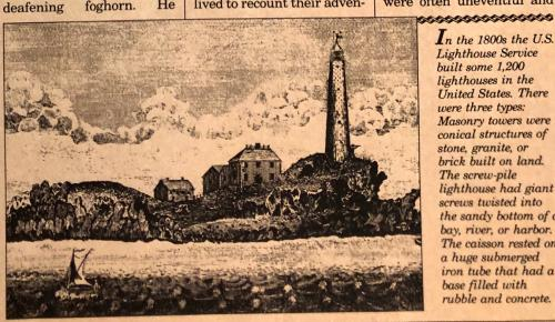
In the 1800s the U.S. Lighthouse Service built some 1,200 lighthouses in the United States. There were three types: Masonry towers were conical structures of stone, granite, or brick built on land. The screw-pile lighthouse had giant screws twisted into the sandy bottom of a bay, river, or harbor. The caisson rested on a huge submerged iron tube that had a base filled with rubble and concrete.
